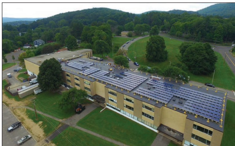
GLEAMING NEW SOLAR PANELS top the roof of Immaculate High School in Danbury. The project, now complete, should save Immaculate 20 percent annually in energy costs.
