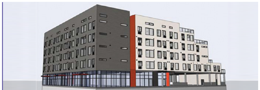
The developers of this 89,000-square-foot complex optimized the building’s original design to qualify for C-PACE. As a result, they were able to drastically reduce their owner-equity contribution.
